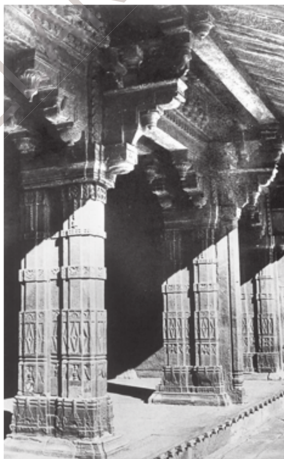
Fig: 22.15 Decorated pillars and struts holding the extension of the roof in Jodh Bai palace in Fatehpur Sikri. They follow the architectural traditions of the Gujarat region.
