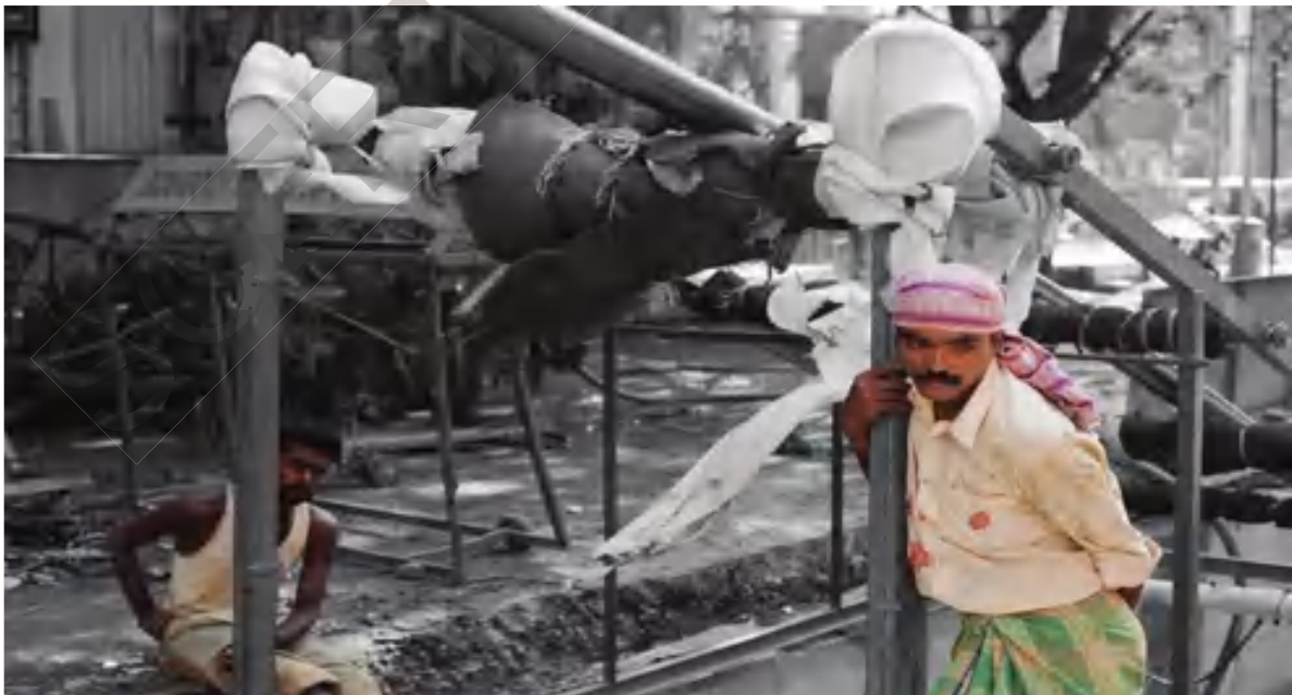
Fig 19.5 Road Laying Work
