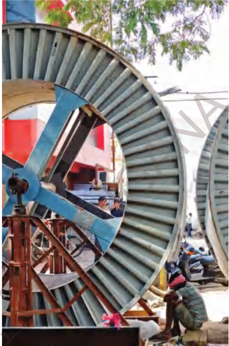
Fig 19.4 Workers laying cables
